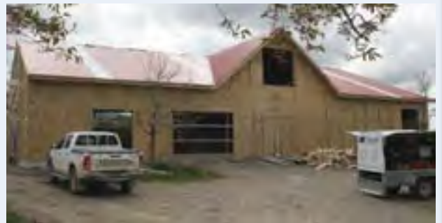
The new shed at Peel Forest is almost complete.
